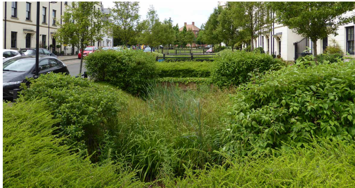
Attenuation basins, swales and landscaped rain gardens will be key elements of the SuDs strategy
